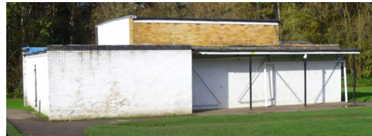
What the pavilion looked like before the roof works
